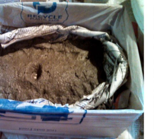
Pack mix heavily (3/4" or more) over the area of the channel, then make drainage hole(s) along the channel.
